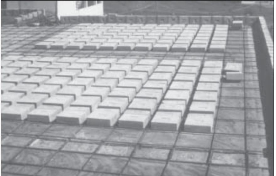
SMB filler blocks with reinforcement
