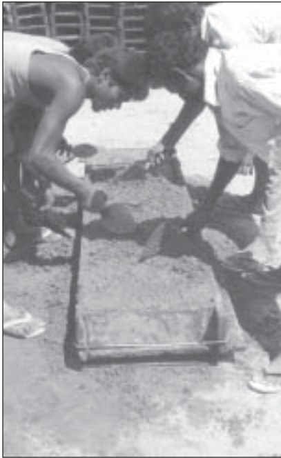
Casting of ferroconcrete channel floor units
