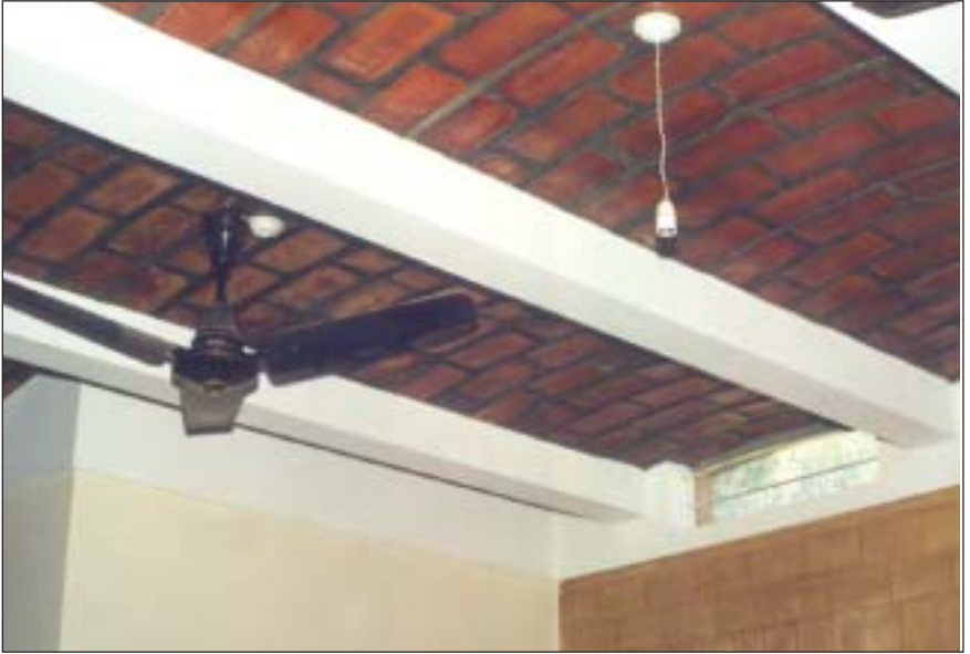
Reinforced tile-work jack-arch roof ceiling
