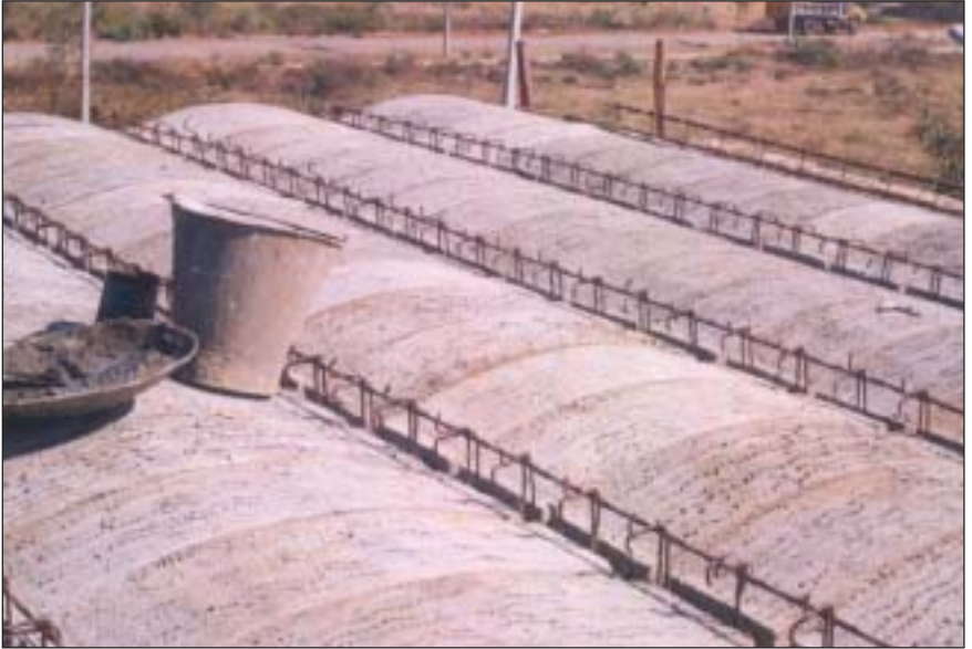
Composite jack-arch roof assembly
