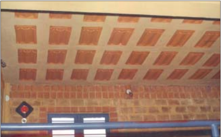
Mangalore tile filler slab roof ceiling
