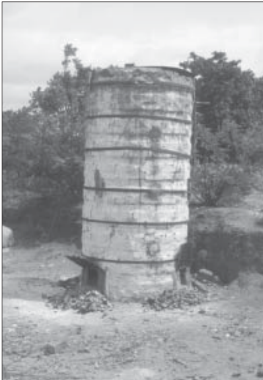
\frac{1}{2} ton capacity lime kiln
