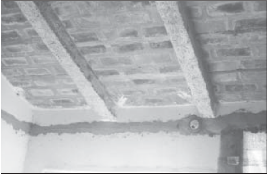
Reinforced brick-work flat panel roof
