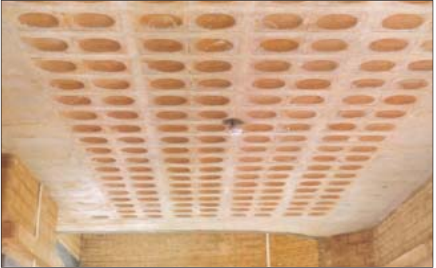
Ceiling of SMB filler slab roof before finishes
