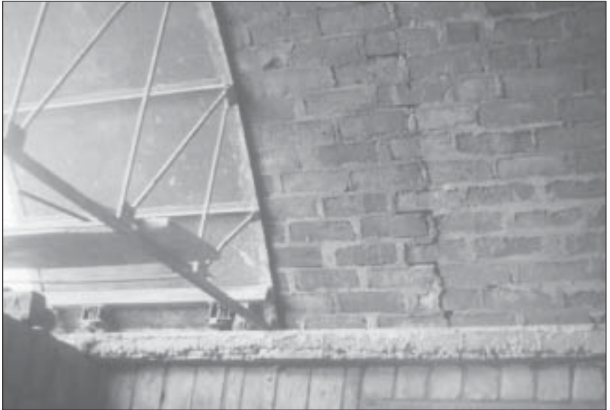
Masonry vault construction under progress
