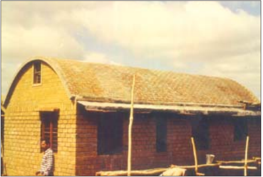
Masonry vault roof
