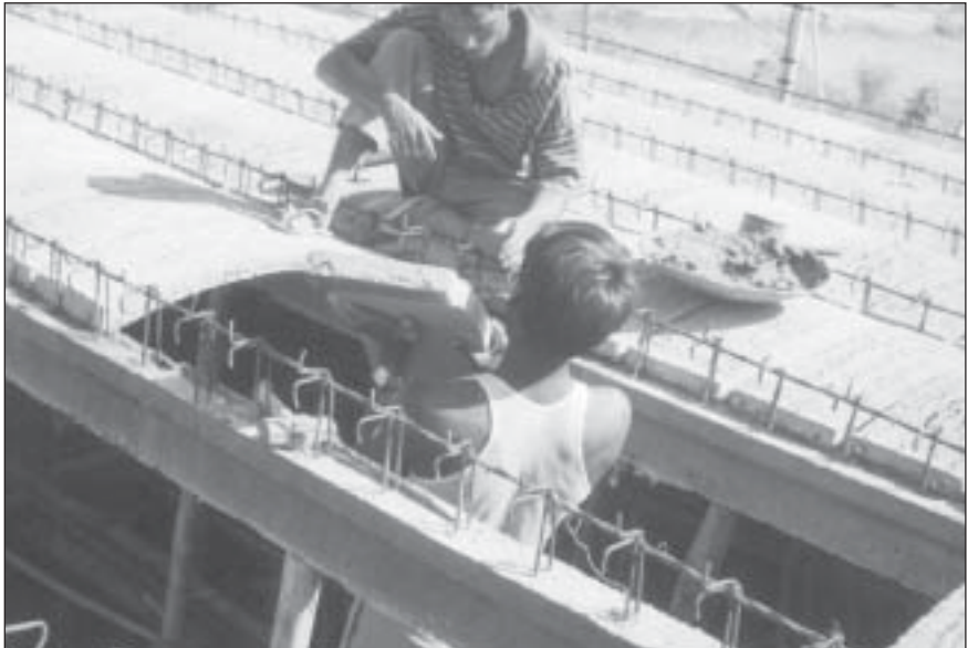
Details of composite jack-arch panel roof
