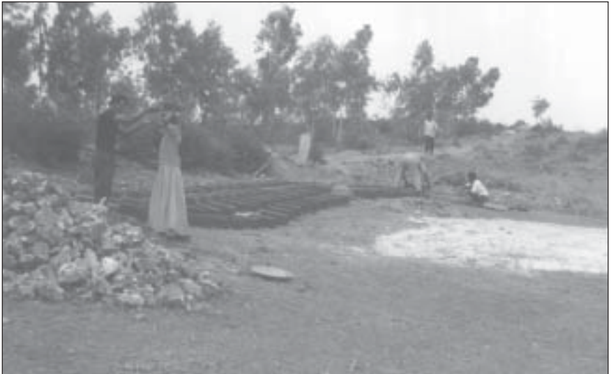
Manufacture of mud concrete blocks
