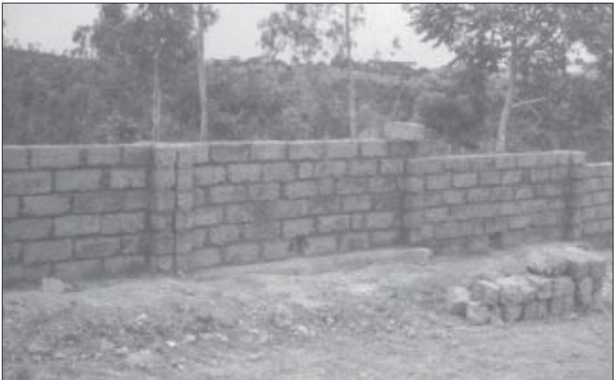
Mud concrete block boundary wall
