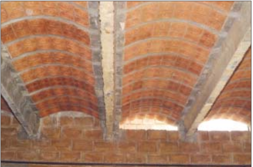
Jack-arch panel roof with decorative clay tile ceiling
