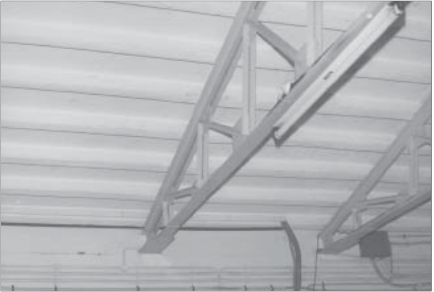
Ceiling of ferroconcrete channel roof
