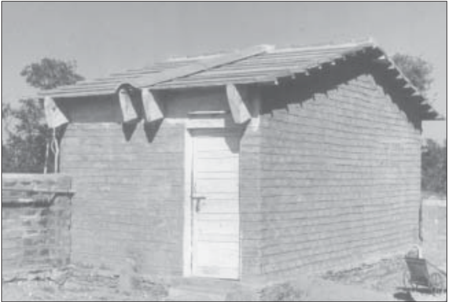
L-beam tile roof
