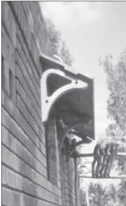
Precast brackets, Chajjas and RB Lintel
