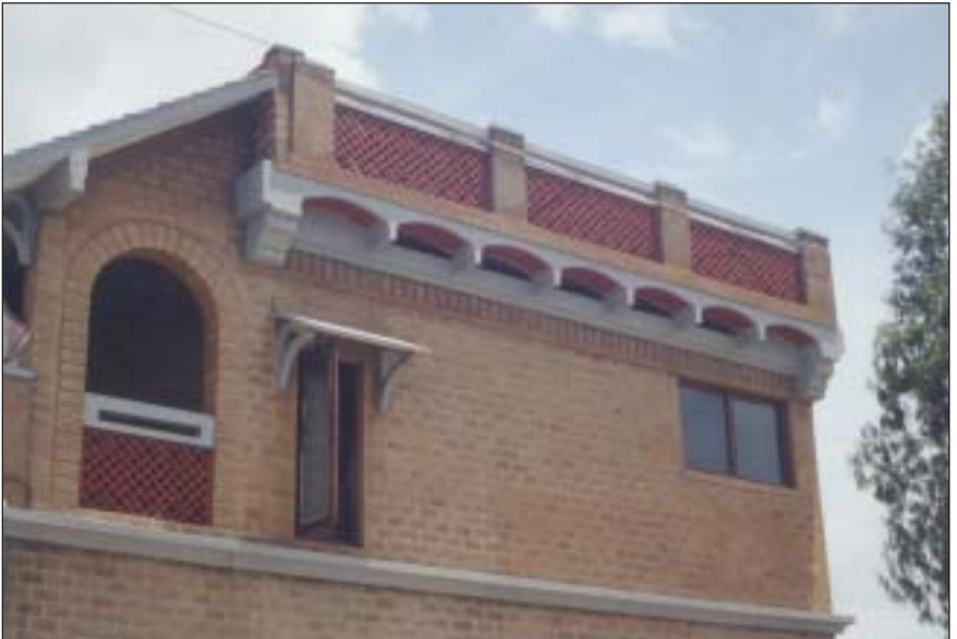
Composite beam panel roof building
