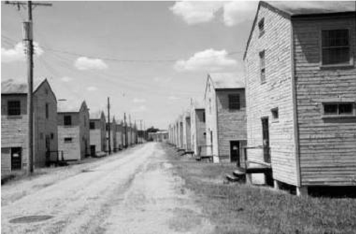
Figure 7. Two-story WWII wood Army barracks.
