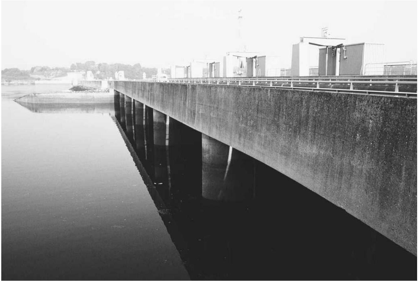
The Barrage de la Rance was the first hydroelectric power plant to generate energy using tidal power. (Corbis-Bettmann)
