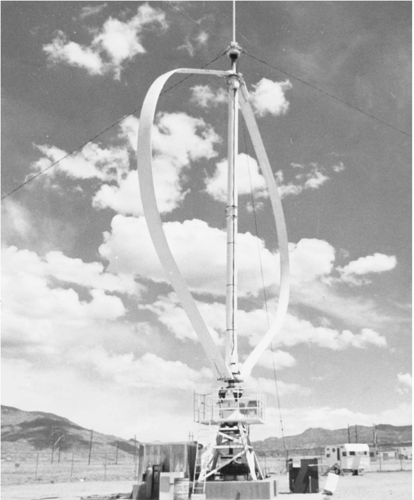
Egg-beater shaped vertical axis wind turbine (VAWT) at the test site at Sandia Laboratories. (U.S. Department of Energy)
