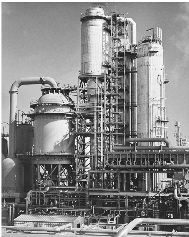
A fluid catalytic cracking unit in Joliet, Illinois, converts heavy components of crude oils into high octane gasoline and distillates. (Corbis Corporation)
