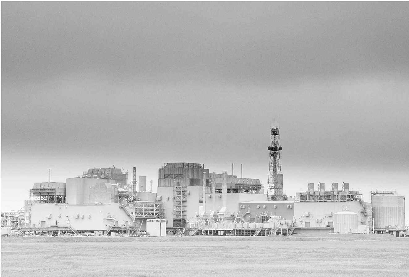
Prudhoe Bay Oil Field. (Corbis Corporation)
