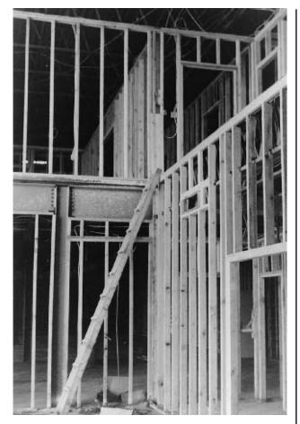
Fig. 12.1.11 A view of framing for the first- and second-story offices of a plant, with a roof beam and the steelwork supporting the second floor visible. (Source: VMA, Inc.)
