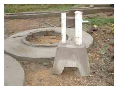
The guide box at the bottom of the well.
