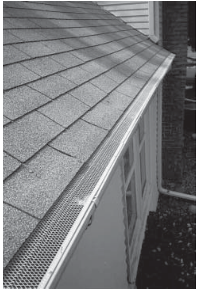
One example of a flat screen over the gutter to keep large debris out of the tank. A problem with gutter screens is that they require a lot of maintenance to keep leaves and debris from piling up and blocking the screens. Also, dirt on the leaves can still be washed into the storage tank.
