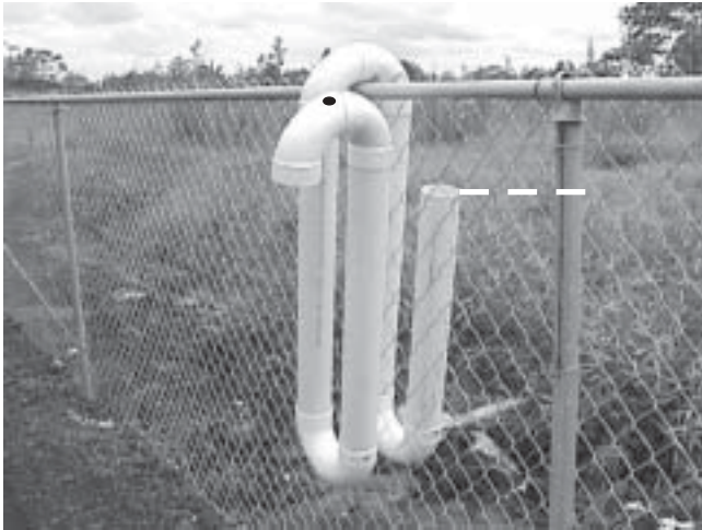
An overflow device to keep the water level as indicated. Pipe on the near side of the fence hangs outside the tank. A hole atop the elbow in the foreground is needed for proper function, but if a T-joint is used, the hole is not needed.
