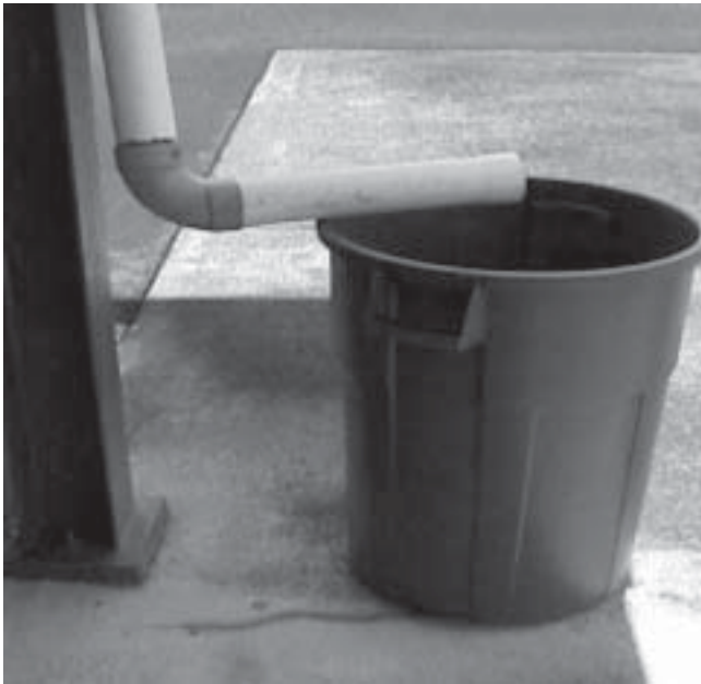
Water collected and held in containers that haven't been approved for water storage can be deadly. Plastic garbage containers, for example, can contain toxic dyes and biocides that could leach into the water.
