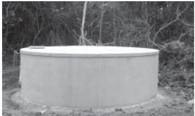
Ferroconcrete tanks, also known as ferrocement tanks, are new to the local market and growing in popularity. Like solid concrete tanks, they can be designed into a home's structure.
