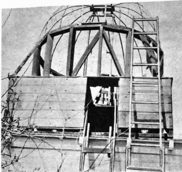
PARTIALLY COMPLETED observatory showing 2x4 framework and skeleton for dome.
