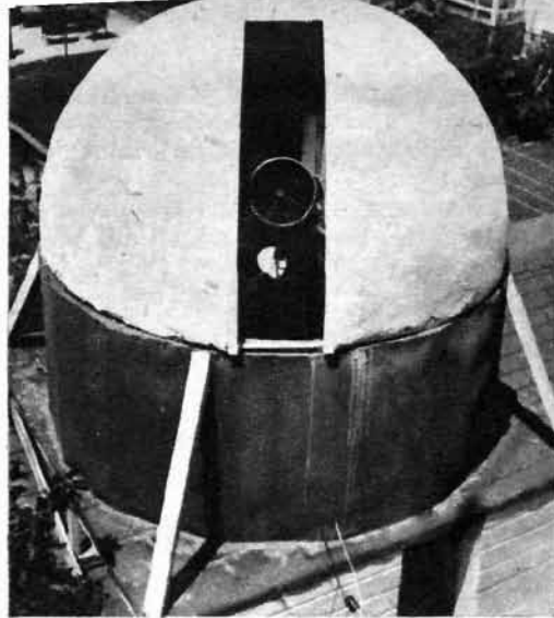
DOMES is finished with a half-inch thick coat of cement. Telescope is a Newtonian.
