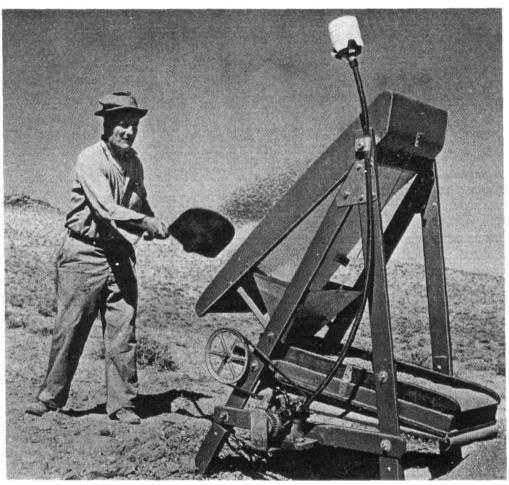
The sifting operation can kick up dust, so to protect the engine, add a heavy-duty air cleaner above the trommel. The drywasher can be hand-cranked, so the engine is optional
