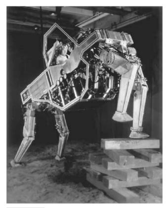
FIGURE 2.1 This quadruped from General Electric was controlled by a human operator who sat inside it. The robot was developed in the late 1960s under a contract with the U.S. government. Photo courtesy of General Electric.
