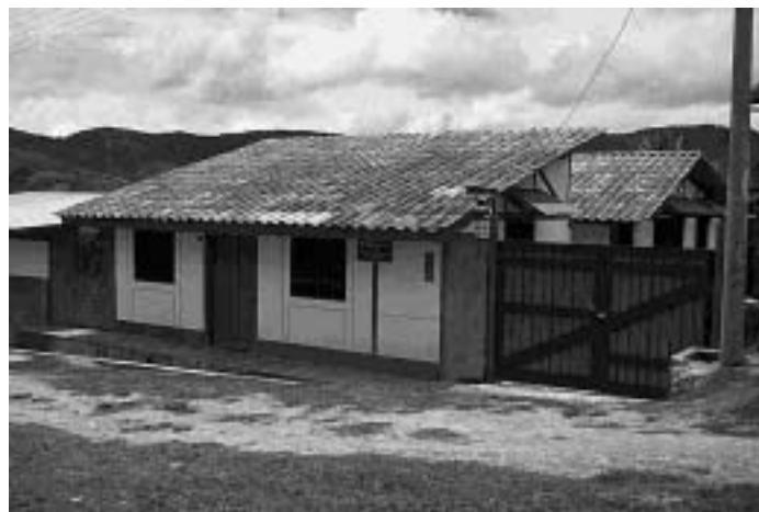
Figure 11: Improved quicha building in Jepelacio ©ITDG/Lucky Lowe
