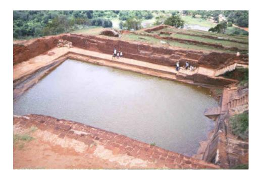
Figure 1: Sigiriya, Sri Lanka. This reservoir cut into the rock was used centuries ago to hold harvested rainwater.
