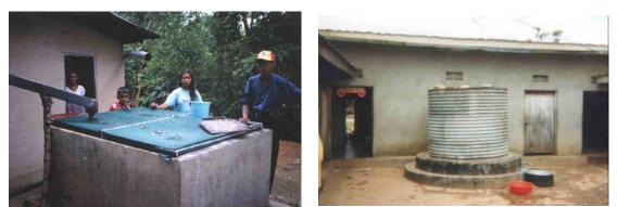
Figure 3: a) An owner built brick tank in Sri Lanka. b) A corrugated iron RWH tank in Uganda.
