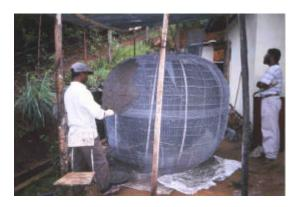
Figure 14: a) One of the 10 legs used to form the skeleton frame. b) The skeleton frame being rendered.
