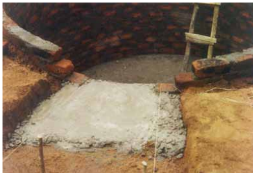
Figure 7: Concrete base for the inlet construction
