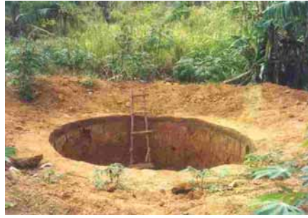
Figure 3: Pit for the tank construction
