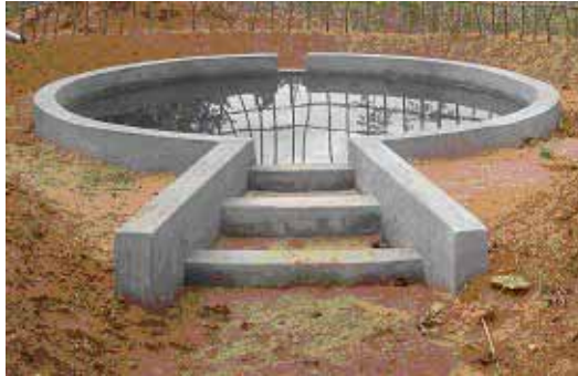
Figure 14: After the Completion of the Rainwater-harvesting tank
