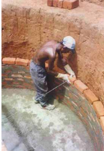
Figure 5: Wall construction of the tank on the concrete base
