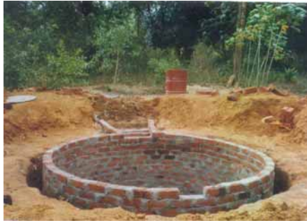
Figure 11: Completed tank before plastering
