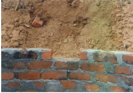
Figure 10: Outlet of the tank
