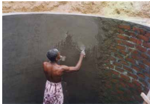
Figure 12: Plastering the tank
