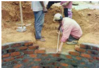
Figure 6: Measurement taken for the inlet construction
