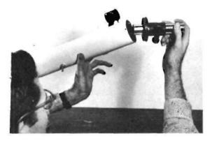
Rack-and-pinion eyeptece mounting comes next: it is inserted in rear end of tube, anchored in place by machine-screws through already drilled holes.
