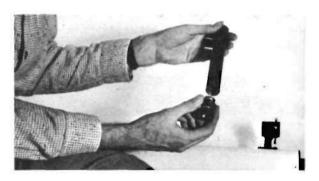
Eyeplece of small finder-scope is unscrewed so that finder-tube may be inserted through its mounting bracket, fastened to the aluminum telescope-tube.
