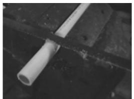
Figure 8-2: Cutting the CPVC pipe with a hack saw to the desired length.
