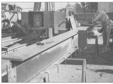
4.5 Virtually any building over single-family-home size requires structural steel in its construction, and that requires arc welding. Here a large beam is being prepared for earthquake retrofit in a public school.
