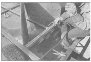
5.32 Gas-shielded MIGs are not made for outdoor work, but as long as you can keep the wind currents away, they work fine. On this driveway utility-trailer project, pieces of plywood are used as wind shields while welding.
