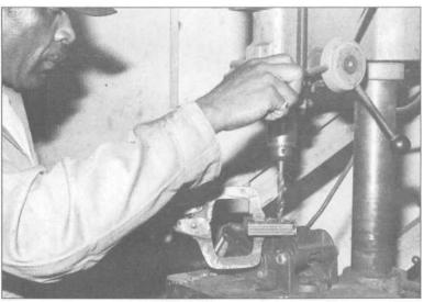
9.21 After flame-cutting, torching or plasma-cutting your plates, sand the edges smooth and stack them together with a vise-grip clamp. You can drill all four plates at the same time, saving time and ensuring that all have the spring-bolt holes in the same place.
