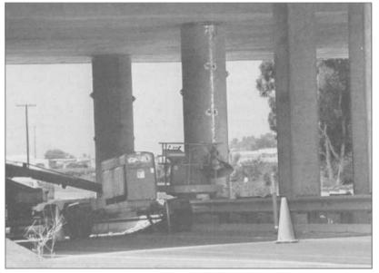
1.4 Under the center bridge column here are a welder (a machine) and a weldor (a person). He is welding up steel enclosures for the concrete columns, to retrofit more strength in California bridges to meet newer earthquake codes.
