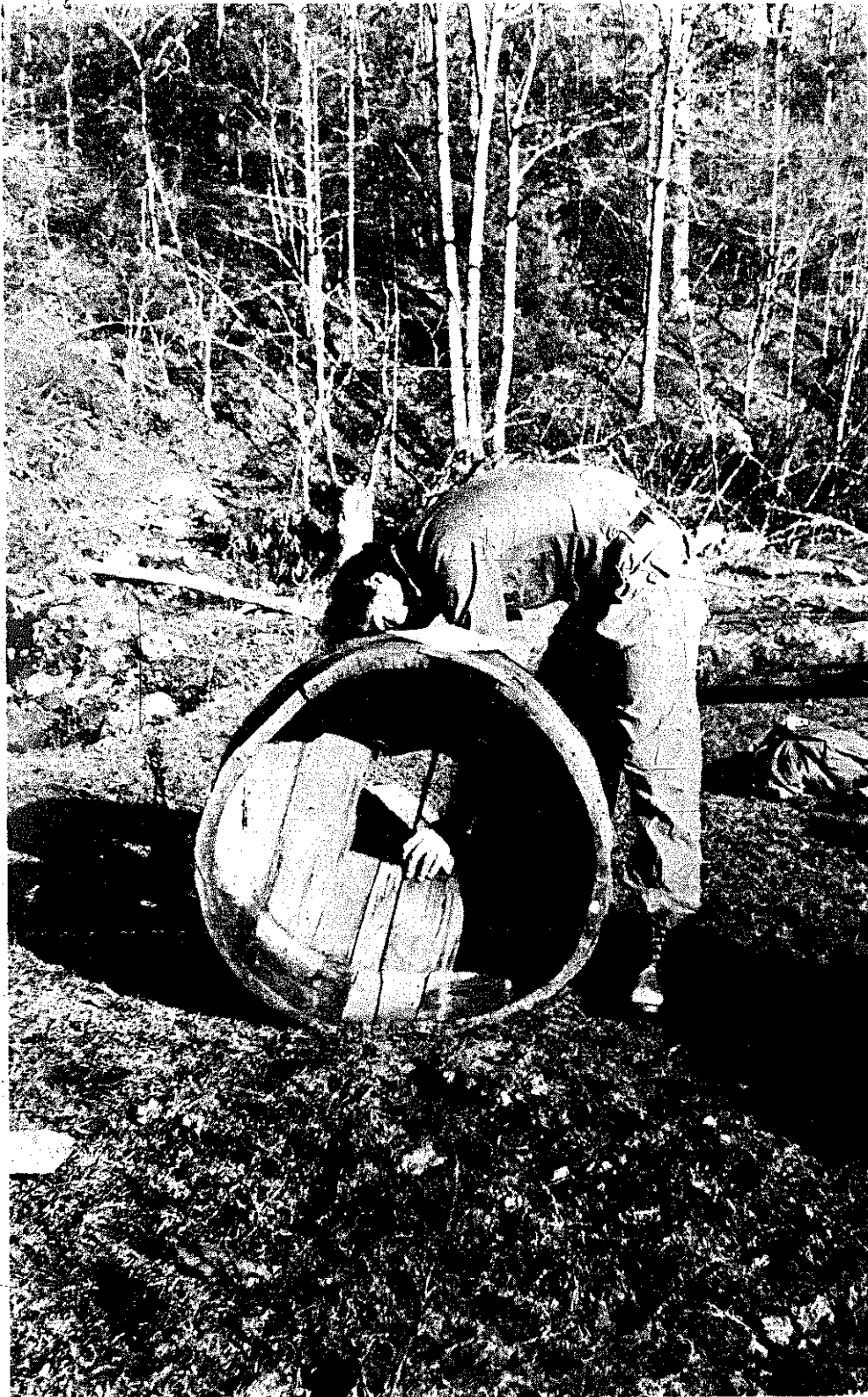
PLATE 167 Ken, Kistner measures the wooden housing that fits over the top of the runner rock. Corn to be ground is poured in a hopper which fits in the central hole visible at Ken's left hand.
