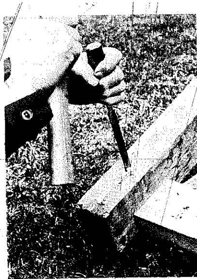
PLATE 169 After the bottoms of the pegs are sawed off flush, Tedra splits the bottom of each peg. Then he drives a wedge into the split to make the peg bind firmly in the hole.
