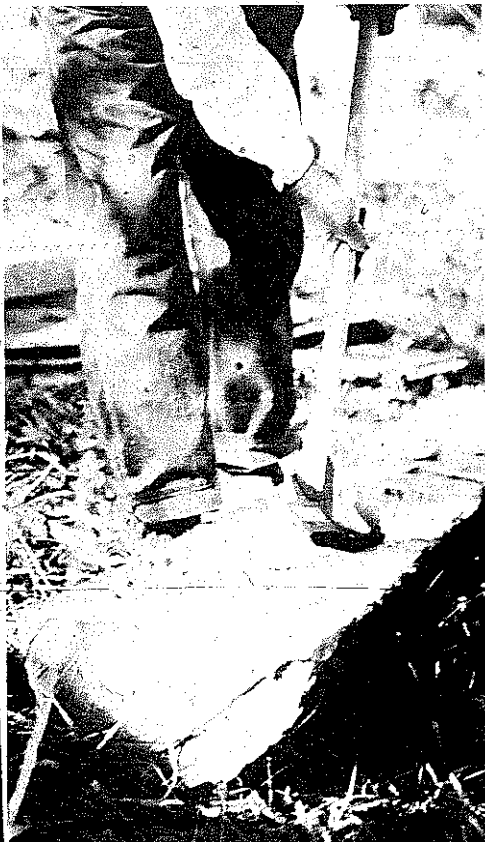
PLATE 406 Millard first splits the poplar log in half and hews the inside smooth.
