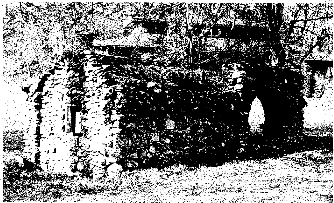
PLATE 334 Point A, view of Hambidge springhouse.
