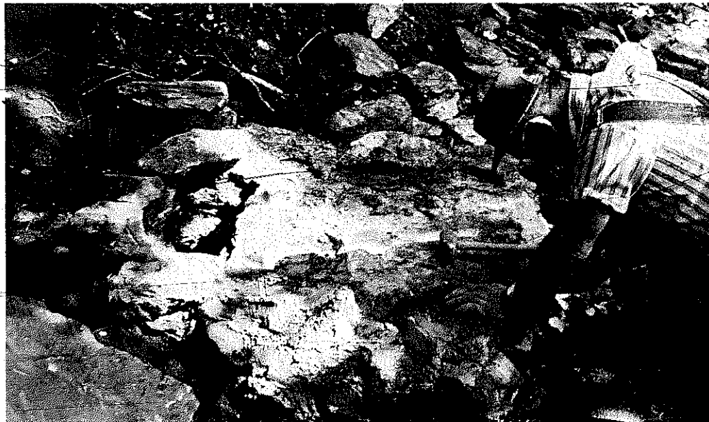
PLATE 430 The hole left at the back of the platform is for the flames, which will come up from the firebox below and wrap around the still, heating the contents to a boil.
