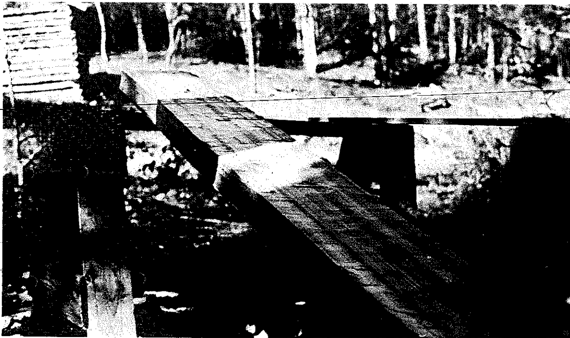
PLATE 410 The finished beam.
