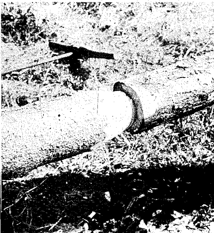
PLATE 314 The tapered end of one pipe fits into the concave end of the next. Just before the pipes are locked together underground, a rag is wrapped around the joint to minimize leaking.
