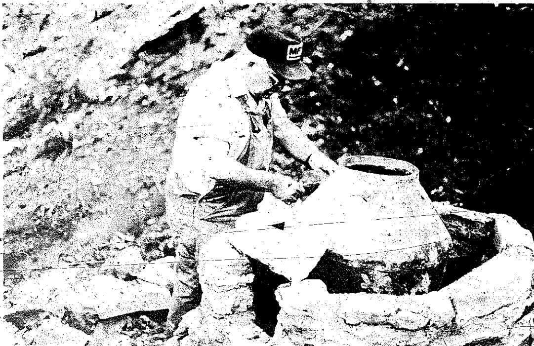
PLATE 438 Next Buck set flat rocks in place around the cape to form the top of the furnace.
