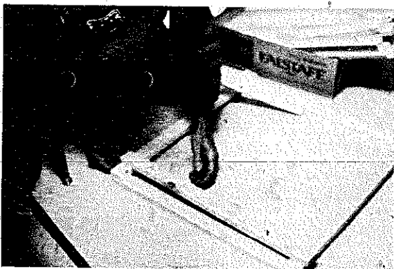
PLATE 219. Lawton begins the trap by laying two boards (24" x 3/4" x 1 1/2") parallel about 22" apart. He then lays two more boards across these to form a square.
