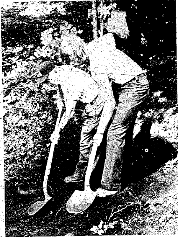
PLATE 427 Here Buck and Joey smooth up the hole, the floor of which will be the floor of the still's firebox.
