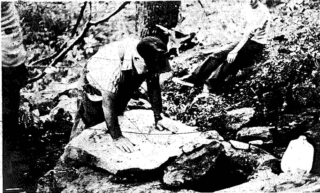
PLATE 429 When the walls of the firebox were high enough (see Plate 431 for measurements), Buck set the large flat rock he had chosen for a bedstone into place so that it spanned the firebox. As it wasn't quite long enough, he set a second, smaller rock into place behind it and cemented the two together to make one flat platform for the still to sit on.
