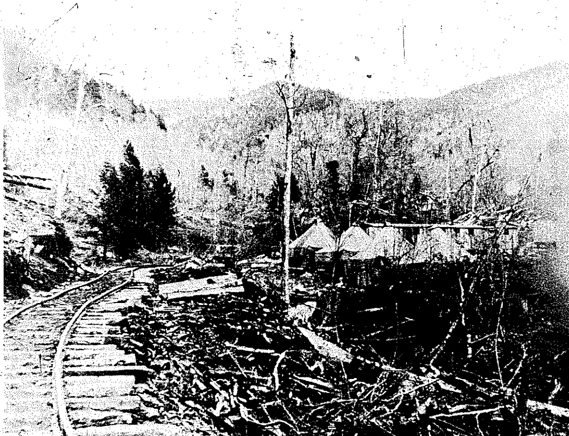
PLATE 287 Another logging camp, this one at the head end of a narrow-gauge railroad line. The dwellings are log sides with canvas roofs. The long, narrow wooden building behind the dwellings is probably the cook shack. An operation like this one might have seventy-five to a hundred men living there at one time. (Photo courtesy of Champion Paper.)
