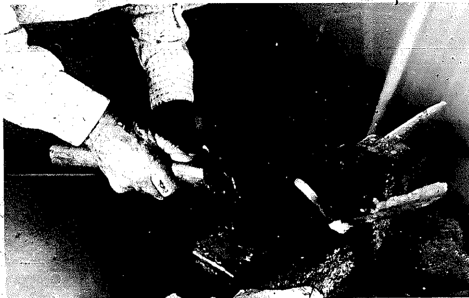
PLATE 93. Making final adjustments in the curve of the shovel handle.
