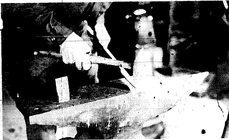
PLATE 63 Finish drawing out the point by hand.
