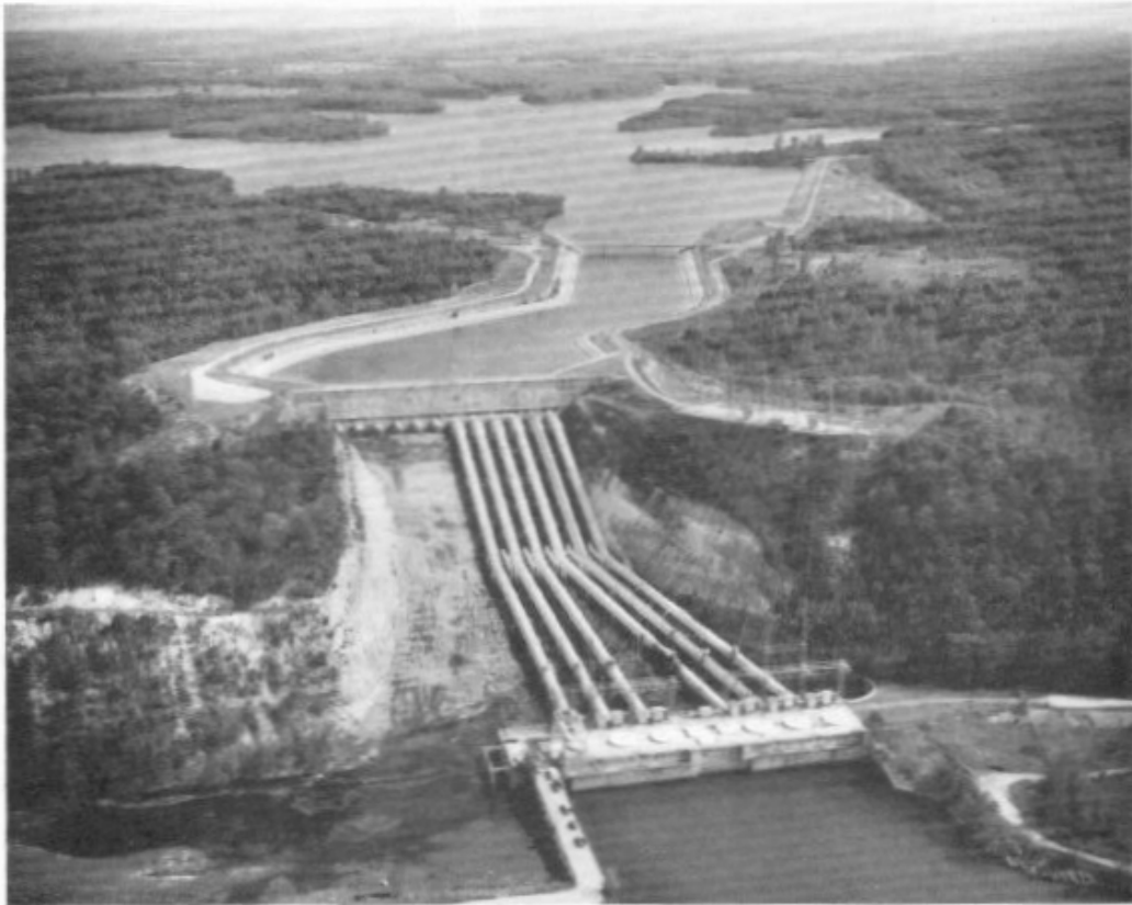
FIGURE 9.14 Salina pumped-storage facility. (Courtesy of Benham-Holway Power Group.)
