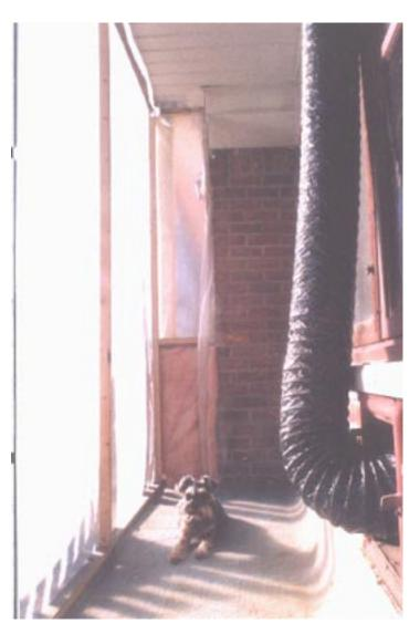
The fan powered duct, through the convenient milk chute, is just an option that I rigged so I can lock up the house and still get the warm air to the inside. When I am around I simply open the door, and the air flows quite well naturally. The pup is not the only one who takes great pleasure in lounging around in the sunspace on a brisk January day.
