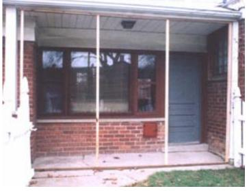
I was concerned, on this house, to not make work for myself when I take this sunspace down at the end of the heating season. There is no caulking or any other attachment, except for the pressure of the fit and two tiny screw holes, up through the vinyl soffit to hold the whole thing in place. It has gone through some pretty tough winds, with no sign of movement. Your detailing will be up to you, and your situation.
