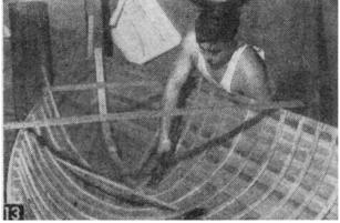
An auto body bucking tool with handle helps in clinching the 1<sup>1</sup>/<sub>4</sub> in. copper clout nails.
