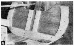
Forward side of transom. Note cheek pieces and strip planks bedded in casein glue around edge.
