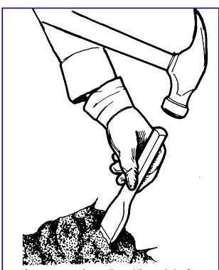
Cut, remove, undercut all crumbling asphalt. Go back to the firm stuff. Use a cold chisel for cuts; wear safety glasses and gloves.
