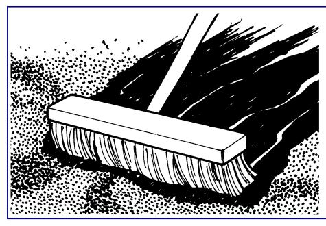
Brush on the sealer with an applicator made for this, or a stiff bristle broom. Don't skimp on the sealer, but don't overdo it either. Work with the brush generally in one direction, removing any puddles of sealer. Let the sealer dry, and then go back over the area looking for thin and missed spots.
