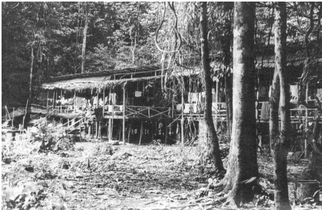
Figure 3.0. The RGS base camp at Long Pala, Mulu N.P. This structure close to the river housed facilities for 30 people, including porters and guides, and was built in 14 days with local labour and dismantled at the end of the expedition.
