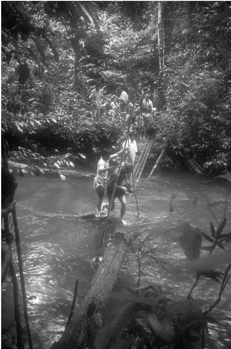
Figure 2.4. River crossing using submerged tree trunk, cut logs, balance poles, and stepping stones. Photo: Bob Hartley
