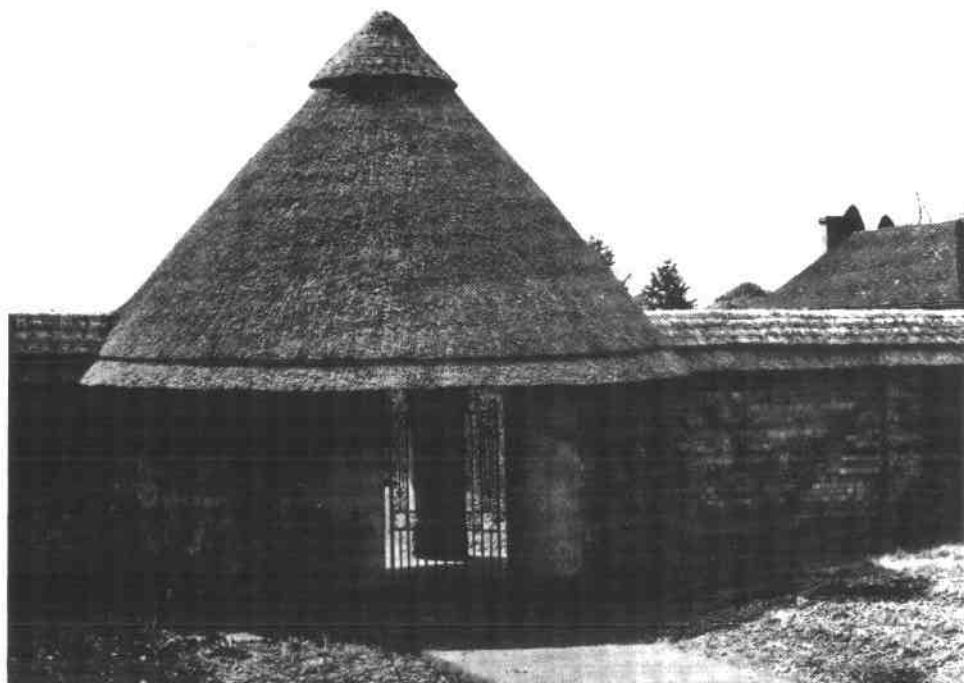
A garden entrance and wall thatched with reed grown in Glamorganshire. Sutton Manor Estate, Sutton Scotney, Winchester, Hants.
