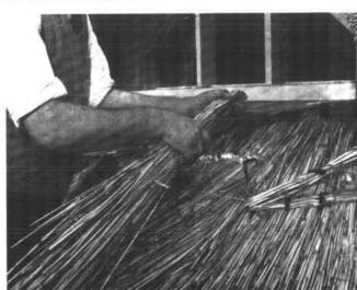
The position of the pattern course, and how it is fixed with twisted bond sparred in is shown.
