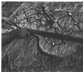
After the first cut round the scallop is made with the small knife, the shears are used to trim the pattern into shape.
