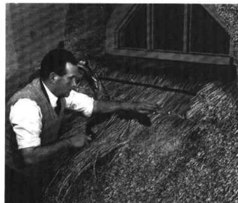
When the whole course is laid it is hooked in with a hazel sway, and for extra strength, a twisted bond is sparred in if desired.
