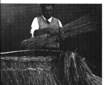
The third and final roll is now sparred down. This not only provides a narrow top but also makes a firm, level base upon which to lay the ridge-course.
