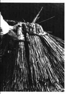
The tufted end is tied in and trimmed and the work of laying the pattern course proceeds.
