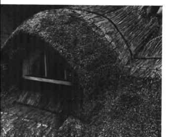
All the eaves-wadds are now tied in over the window. The upward pressure of these wadds is exaggerated by the tilting fillet in the window construction. This pressure, combined with that of the next course, makes a tight eave.
