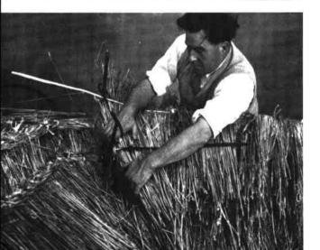
The needle is used as a lever to compress the bunch.
