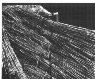
The wadds in the two barges are now joined and those in the centre portion form a small eave for the cap-end.
