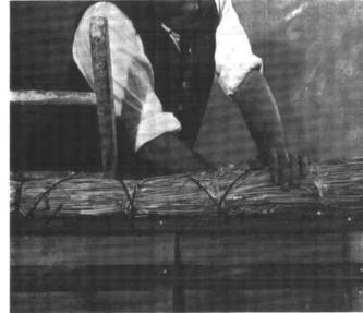
Whilst retaining the tension with the left hand, the cord is passed under the tie, thus locking the stitch.
