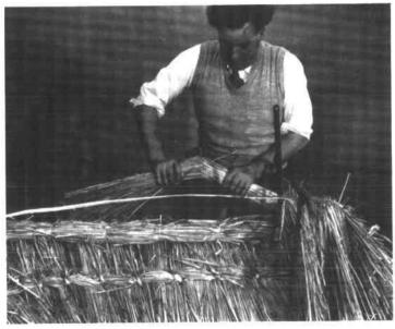
Half of the reed is reversed in order to make both ends of equal thickness.
