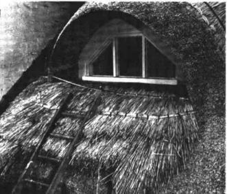
The reed is worked tightly underneath the lead apron and held in position with a temporary sway.
