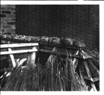
The roll serves the two-fold purpose of (a) providing extra springing to the top course of reed; and (b) a tight base into which spars may subsequently be driven.
