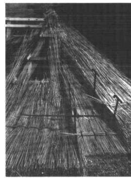
From the vertical position of the centre rafter, the eaves-wadds now turn in the opposite direction, whereupon they join up with the left-hand barge, in line again with the angle of the hip-rafter.
