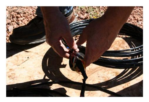
Preparing an explosive charge to 'hydrofract" or loosen or dislodge any debris or corrosion inside an existing well casing. This explosive material is made in 25 or 50 foot lengths and has a blasting cap to start the explosion. Believe it or not, you cannot hear the explosion, since it is deep underwater. The bottom photo is the remains of the explosive charge. This procedure will usually increase well production.
