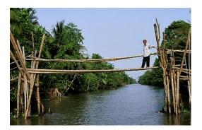
Simple bamboo balancing bridges, with handrails.
