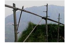
Bamboo pipes that carry water downhill, and support poles (made from small trees).
