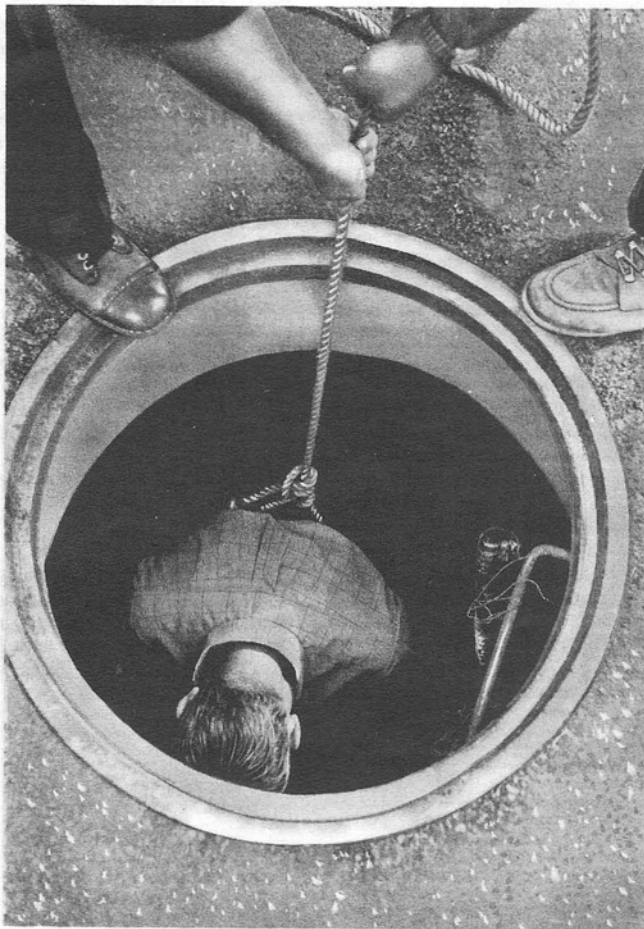
Fig. 1—Rescuer's Position at the Manhole
