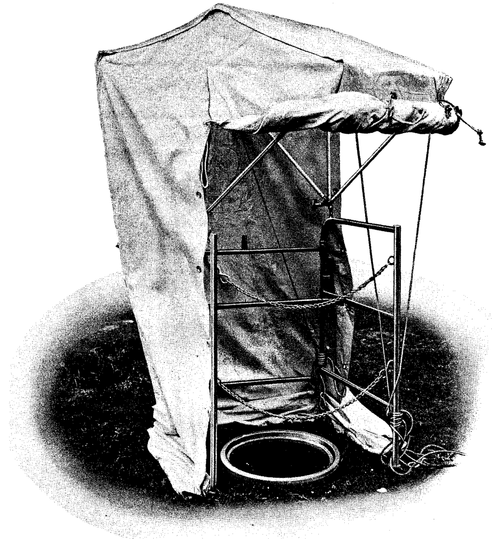
Fig. 11—D Workman's Tent Placed on Manhole Guard
