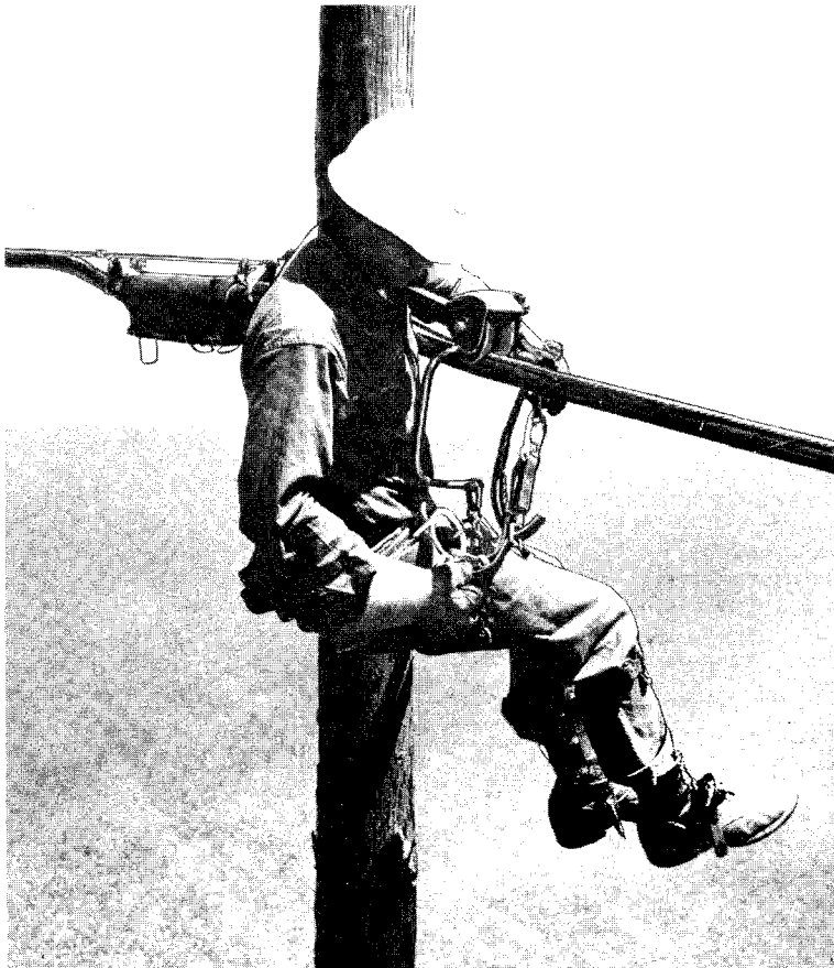
Fig. 3—Attaching Cable Car Straps to Dee Ring
