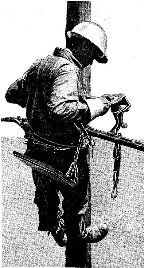
Fig. 9—Placing Car on Strand
