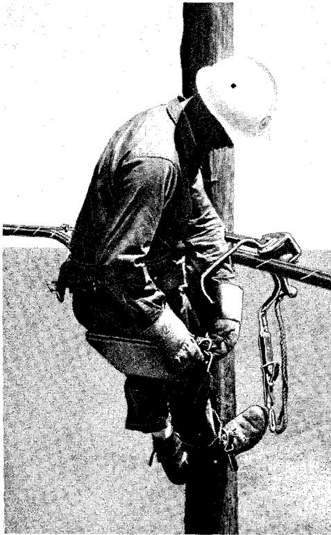
Fig. 4—Refastening Chain on Cable Car Seat
