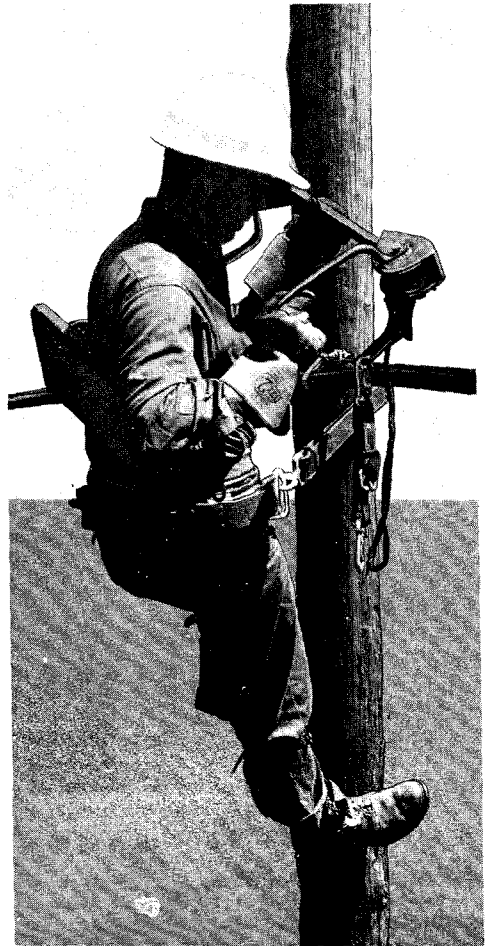
Fig. 2—Passing Cable Car Seat Behind Head
