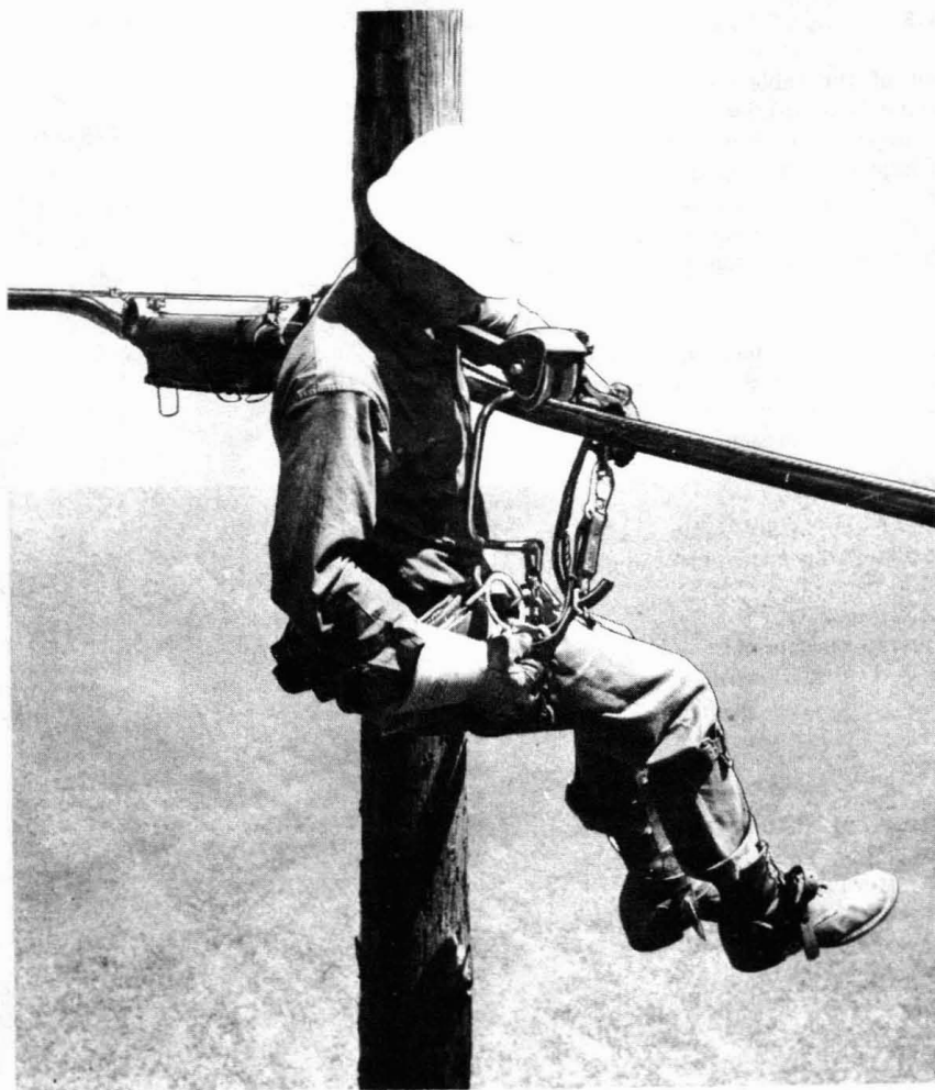
Fig. 3—Attaching Cable Car Straps to Dee Ring
