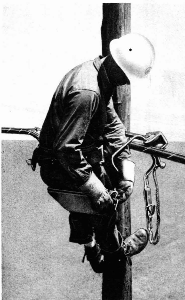
Fig. 4—Refastening Chain on Cable Car Seat
