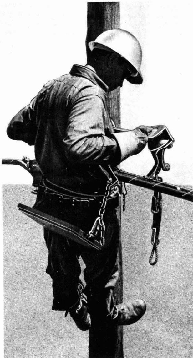
Fig. 9—Placing Car on Strand
