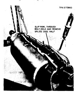
Fig. 6—Removing Outer Splice Case Half
