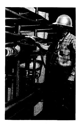
Fig. 20—Locating a Leak Using Hand Probe Method
