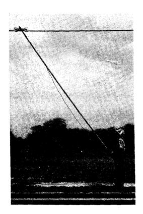
Fig. 18—Locating a Leak Using Trolley Method
