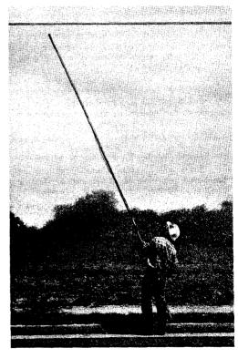
Fig. 19—Locating a Leak Using Wand or Pole Probe
