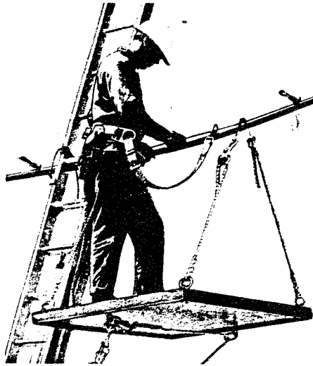
Fig. 8—Method of Using Safety Strap When Using Other Than a D, E, or F Belt
