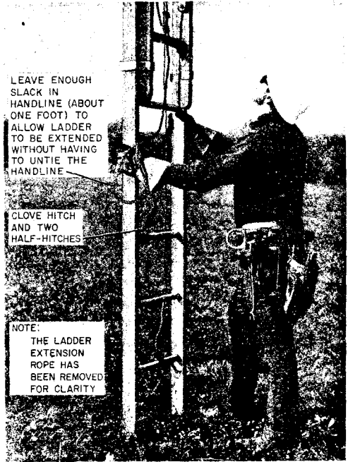
Fig. 42—Method of Securing Handline
