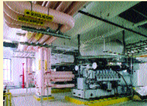
8 Megawatts of new emergency power.
