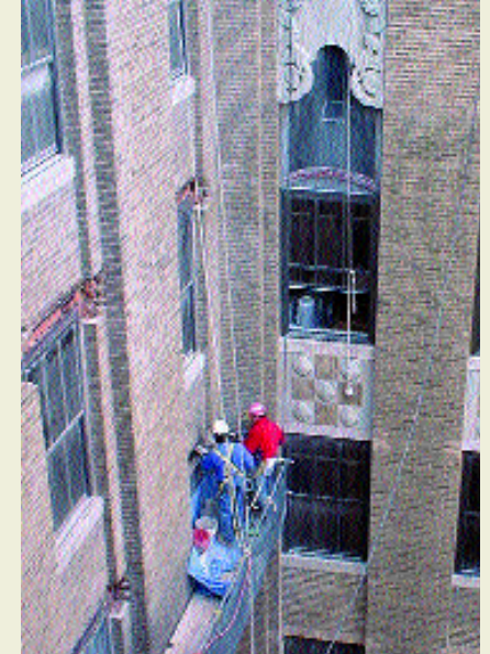
Replaced 1500 landmark windows.
