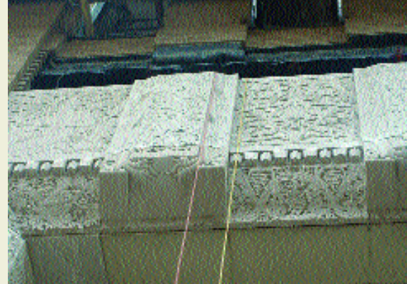
Reconstructed over 45 tons of ornamental limestone.
