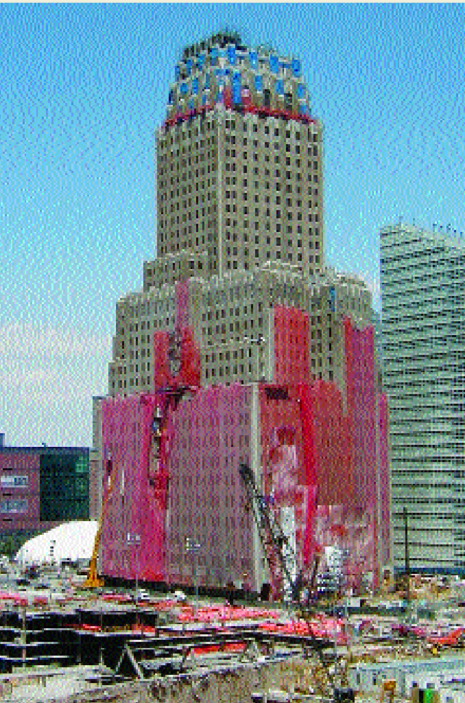
Over 1 acre of new roofing on 20 separate roofs.
