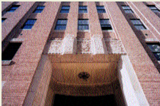
Replaced 475,000 face brick.
