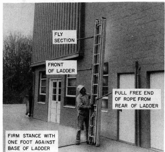
Fig. 23—Preparing to Extend Fly Section
