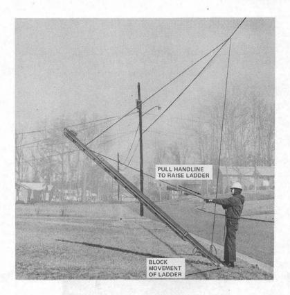
Fig. 18—Ladder Partially Raised
