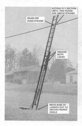
Fig. 21—Ladder in Working Position
