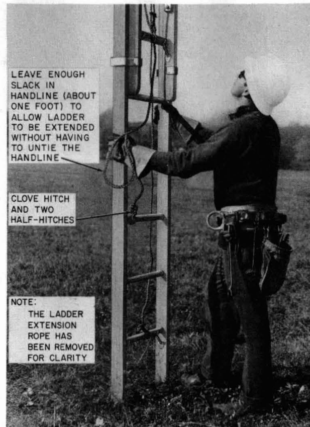
Fig. 20—Method of Securing Handline
