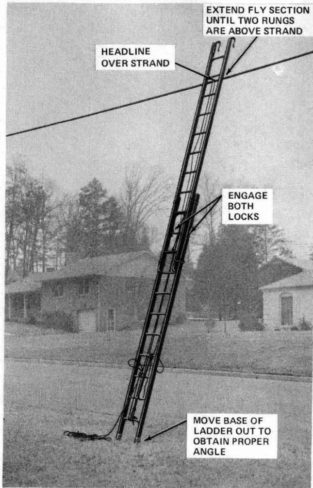
Fig. 21—Ladder in Working Position
