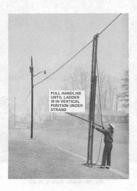
Fig. 19-Ladder in Vertical Position
