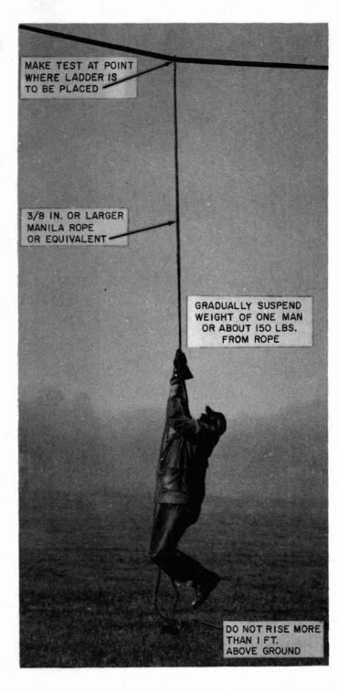
Fig. 2—Testing Strand Prior to Placing Ladder
