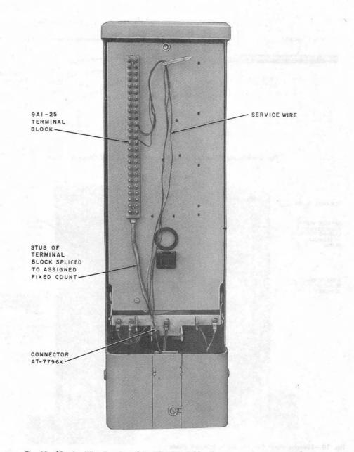
Fig. 12-DService Wire Terminated in PC12/55 Cable Closure-Fixed Count Mode
