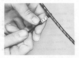
Fig. 2-Placing Tie and Marker
