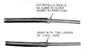
Fig. 26-PRemoval of Metallic Shield
