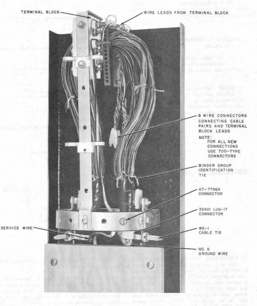
Fig. 16—\$Service Wire Installed—J Cable Closure (Protected)
