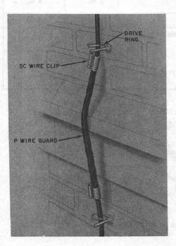
Fig. 3—Crossing Masonry Building Projection
