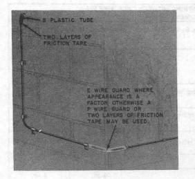
Fig. 2—Use of Tape or E Wire Guard
