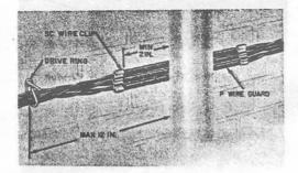
Fig. 7-Block Wires Crossing Behind Pipe
