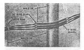
Fig. 6-Block Wires Crossing Over Pipe
