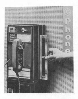
Fig. 10—KS-22473 Leveling Device Being Used to Check Side Alignment
