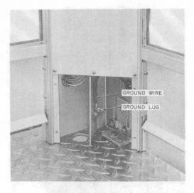
Fig. 6-Grounding Screw in KS-19580 Booth
