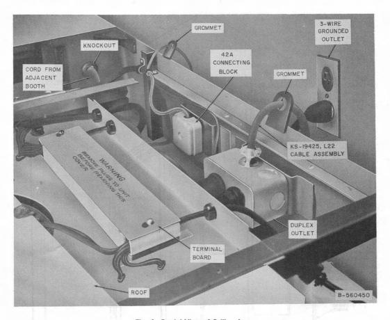
Fig. 6—Partial View of Ceiling Area
