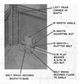
Fig. 7-Booth Anchoring Bracket
