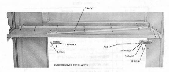
Fig. 23—Installation of Door Track
