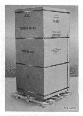
Fig. 16—Kiosk in Packing Case
