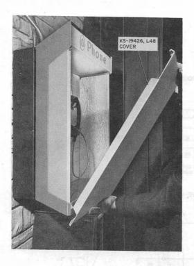
Fig. 24-Installing List 48 Cover
