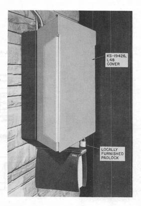
Fig. 25-List 48 Cover Installed
