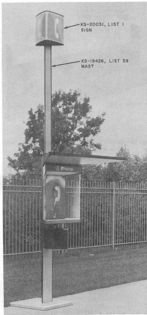
Fig. 18— ⚡ KS-20031, List 1 Sign Installed on KS-19426 Mounting With Canopy ⚡
