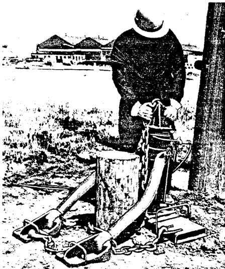
3. ATTACH BRACES TO CYLINDER AND PULLING CHAIN TO BUTT.
