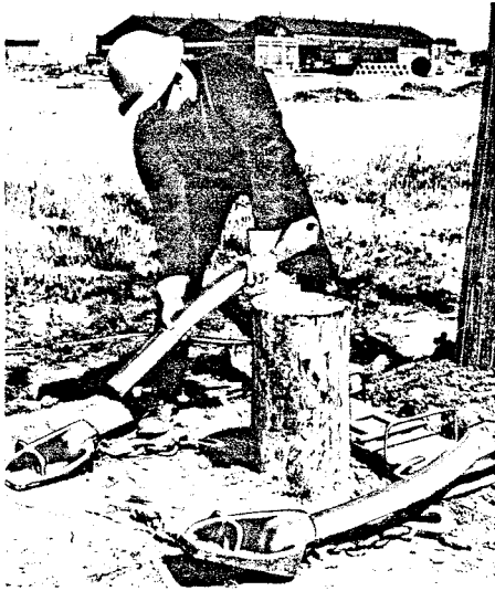
1. PLACE FRAME ASTRIDE POLE BUTT.
